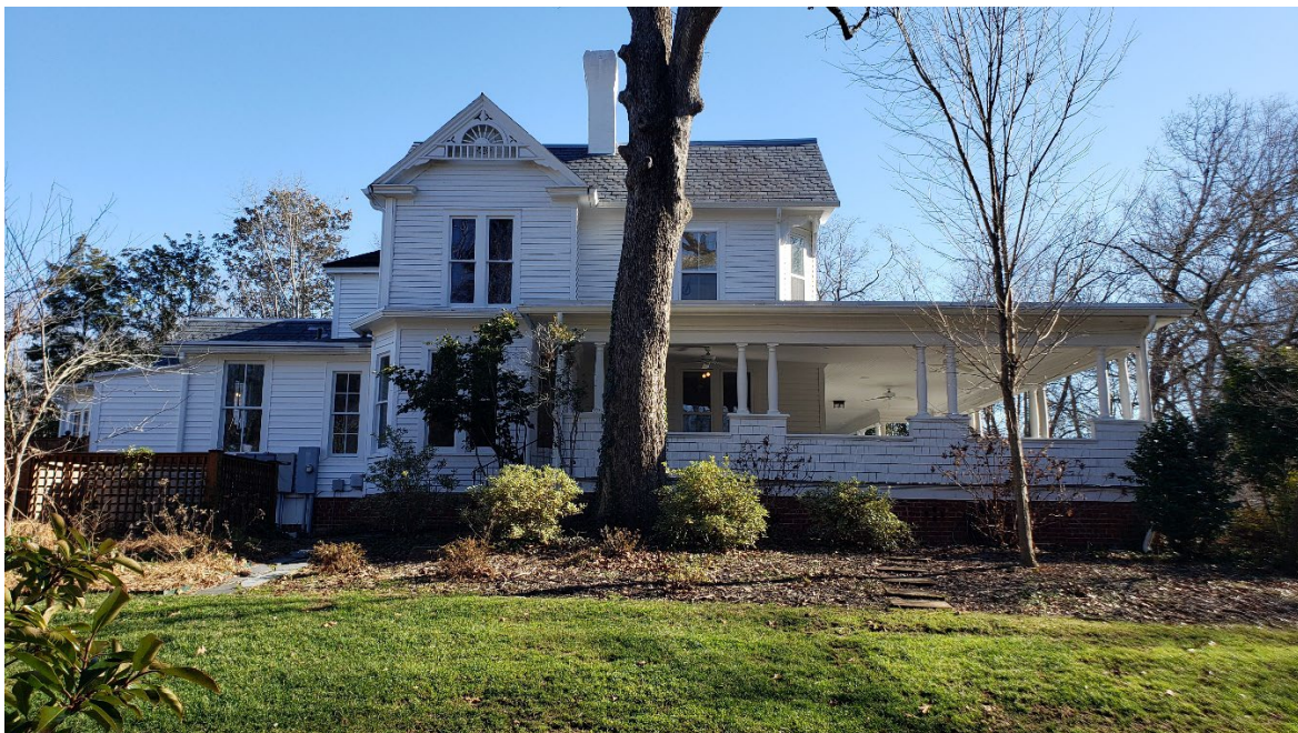
Existing House: View from Left Side
